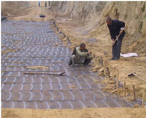
Figure 1: Geogrid pieces held in place
