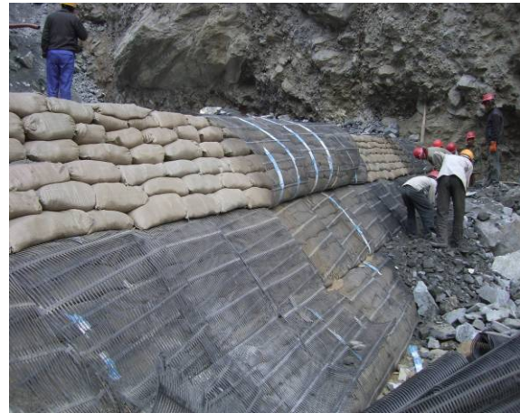
Figure 3: Lifting Geogrid over face
