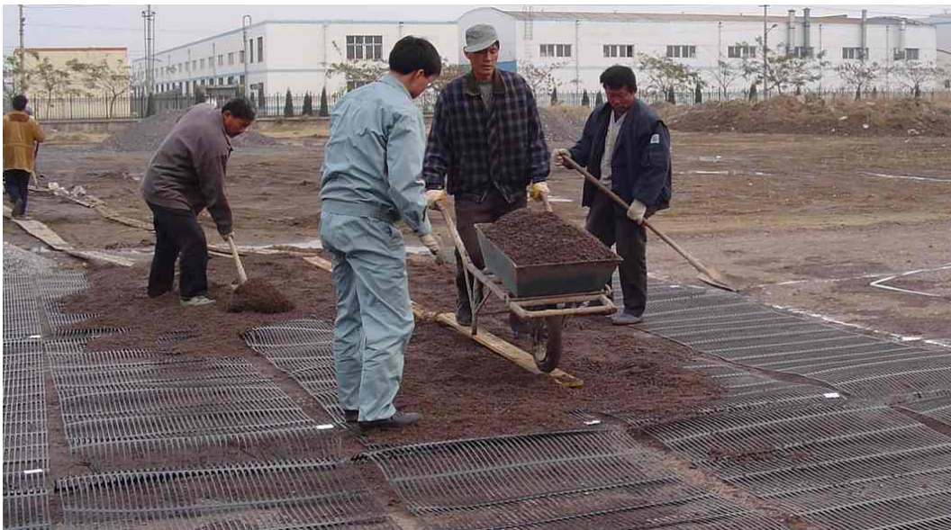
Figure 4: Placement of Fill on Geogrid Samples
