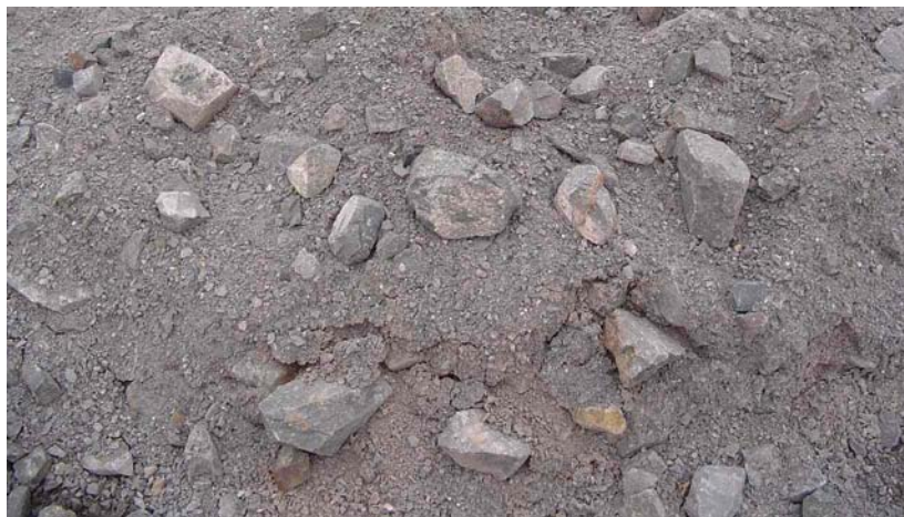
Figure 1: Coarse Fill before Compaction
